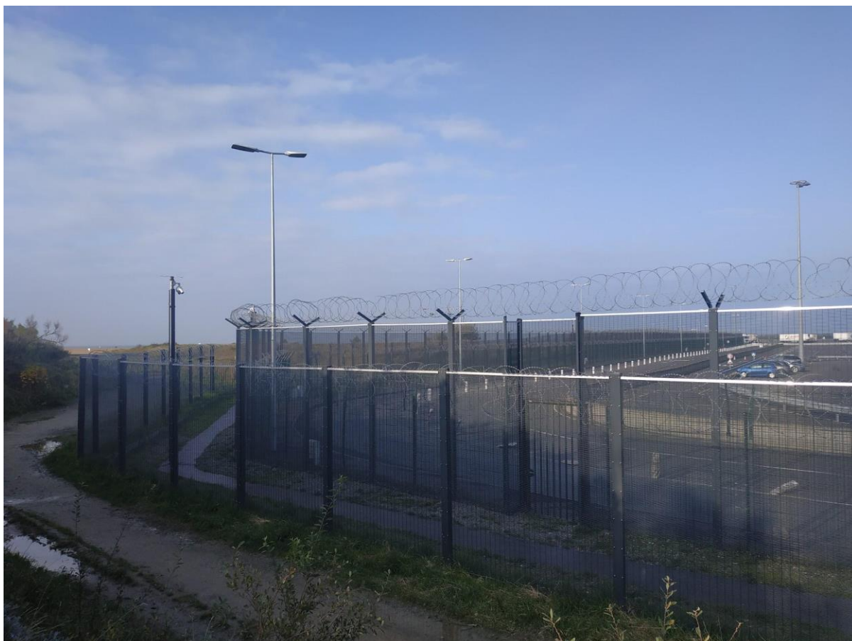
Three rows of fences topped with razor wire and accompanied by surveillance cameras, Ouistréham port (photo credit: Pierre Menzildjian)
